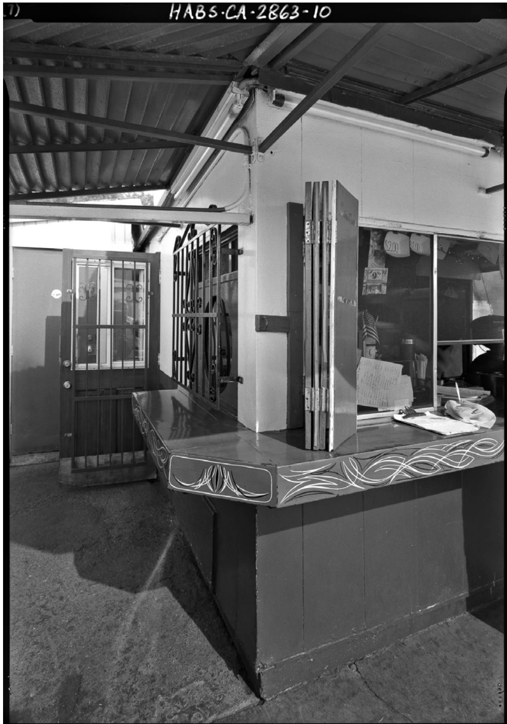
Figure 24. Detail of welded, steel, wrap-around counter and open wood folding doors for pass-through window. February 2010. Source: HABS.CA.2863-10. Photographer: Stephen Schafer.
