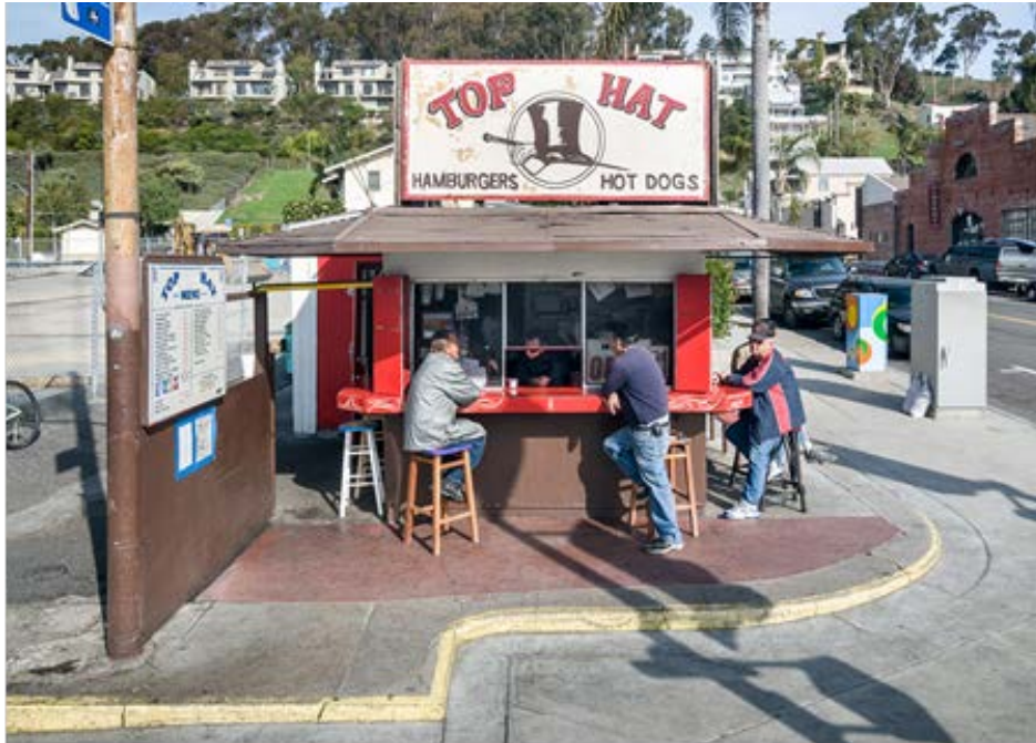
Figure 15. Exterior, oblique view of northeast corner showing steel panels on east façade and Unistrut construction on north façade. Noncontributing shed visible on right. February 2010. Source: Stephen Schafer.
