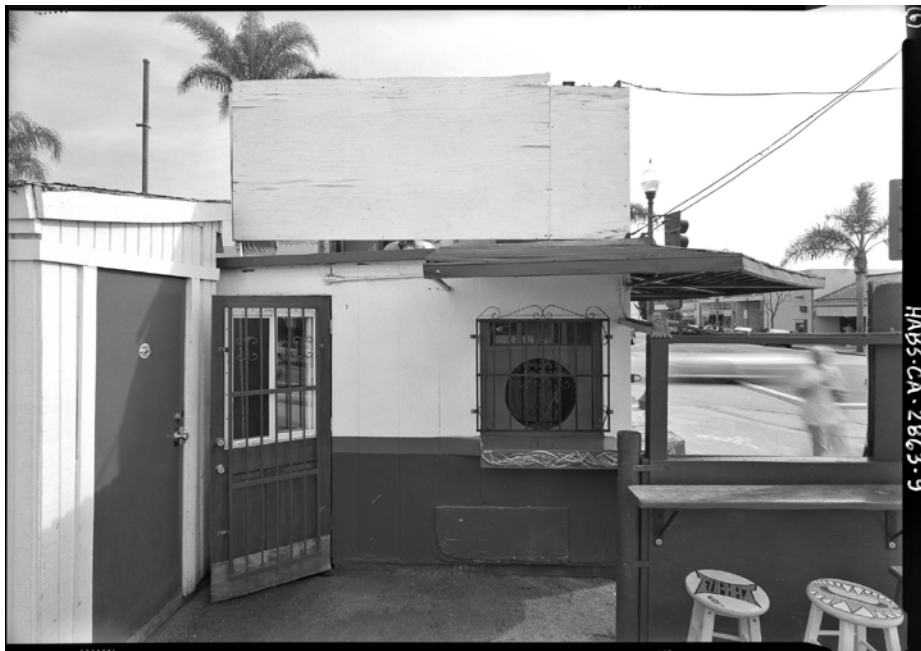
Figure 23. West elevation detail shows steel panel construction. One noncontributing wood storage shed is visible at left. February 10, 2010. Source: HABS.CA.2863-9. Photographer: Stephen Schafer.
